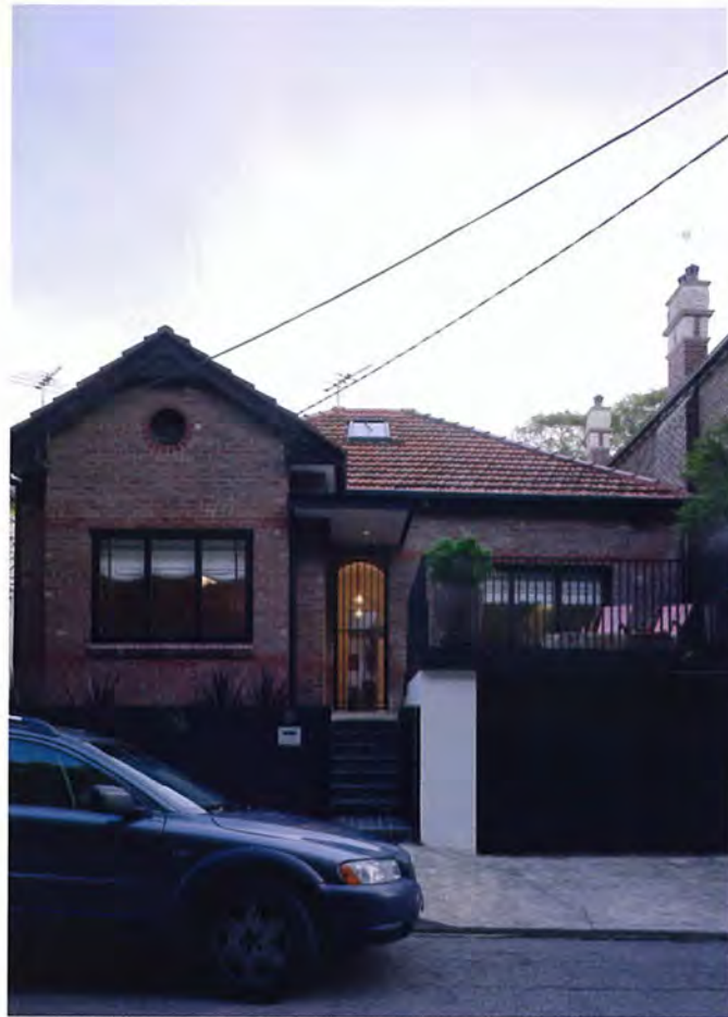
Heritage restrictions required the retention of the Federation facade.
