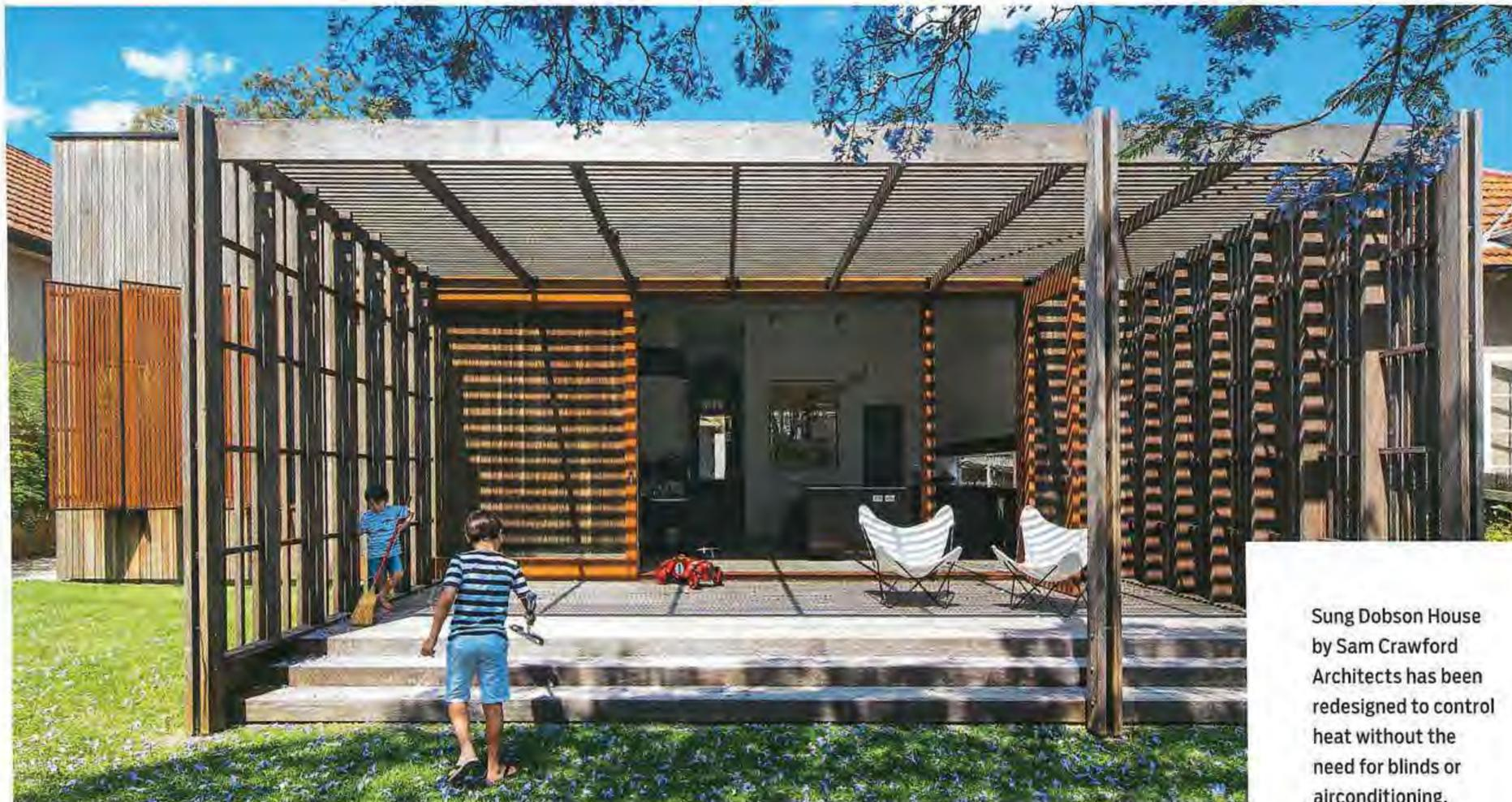
Sung Dobson House by Sam Crawford Architects has been redesigned to control heat without the need for blinds or airconditioning.
